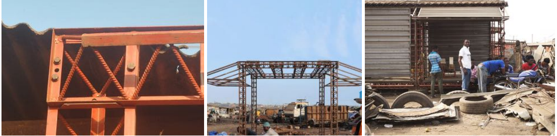
Figures 10 to 12. Agbogbloshie Makerspace Platform in situ construction, 2014
